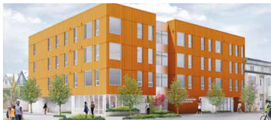
Harvey Rice Heritage is bringing two new affordable housing complexes to inner Northeast Portland, named after renowned artists. This is the Isaka Shamshud-Din Development.
