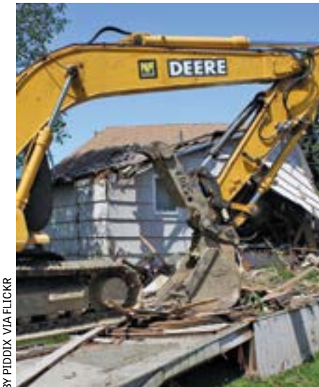
NE Portland house is being demolished
