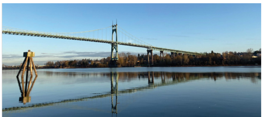
St. Johns Bridge, Portland (Photo/Hunter Young, EPA)
