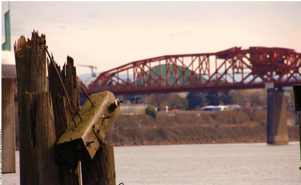
Portland Harbor runs along both sides of the Willamette River, from the Broadway Bridge (pictured) to Sauvie Island
